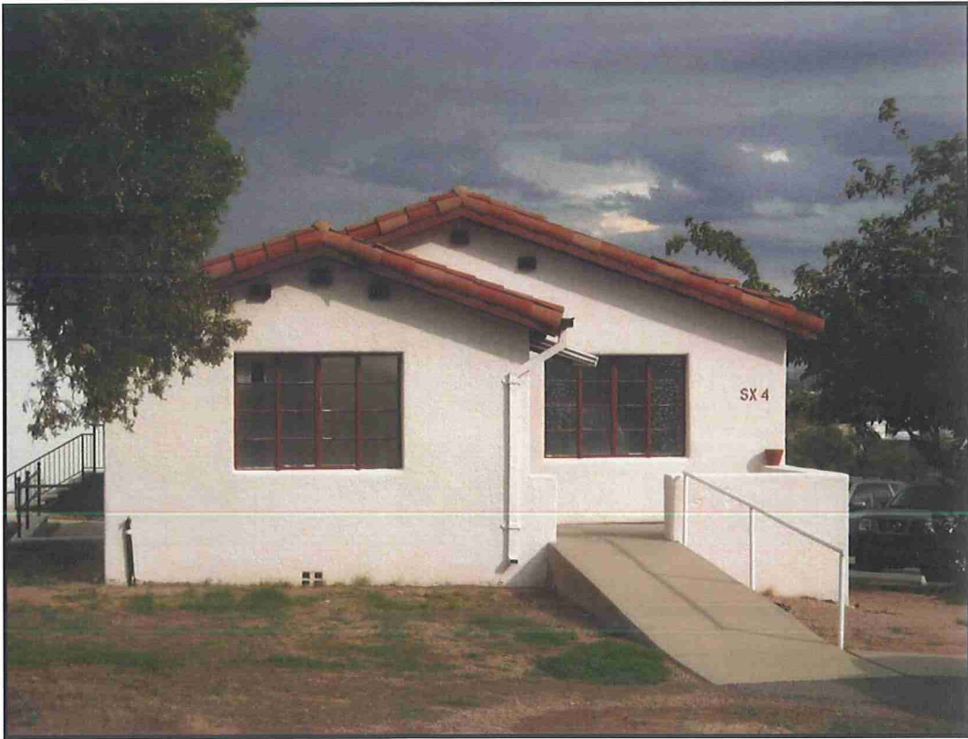
Photograph 40. Former physician housing (San Xavier-4), view facing northwest (2010).
