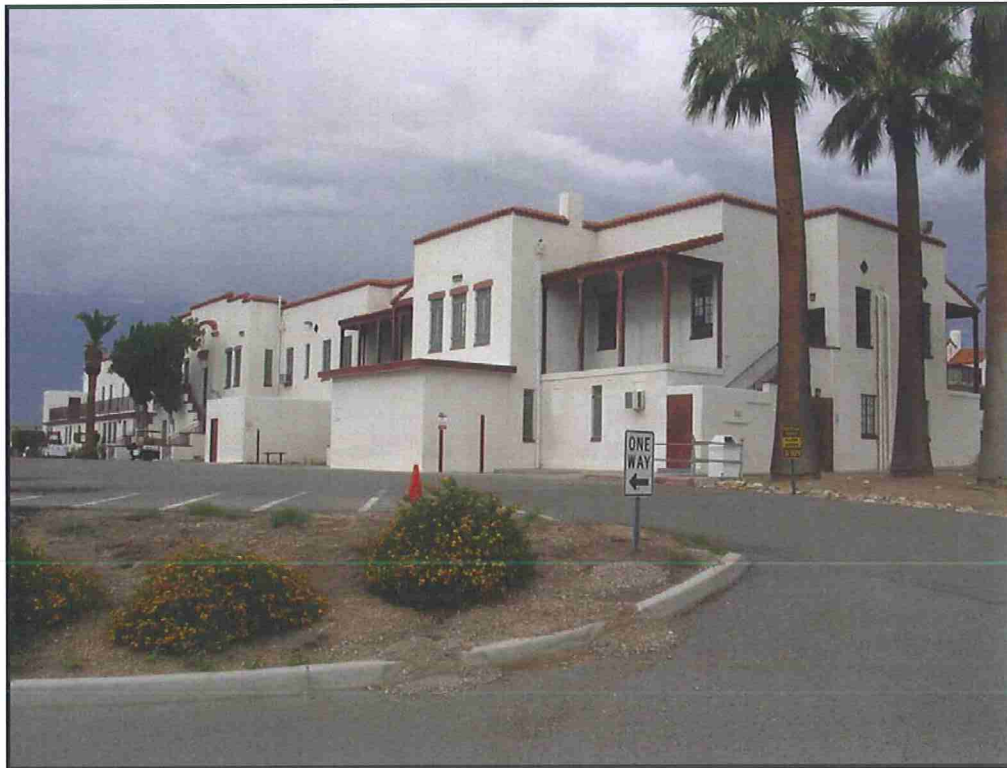
Photograph 37. Main hospital building (SX-1) at the former San Xavier Sanatorium, view facing southeast (2010).
