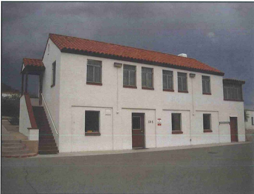
Photograph 42. Former nurse's residence (San Xavier-6), view facing west-northwest (2010).
