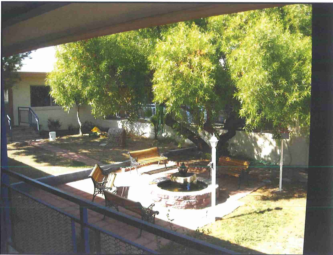
Photograph 59. Interior courtyard view from main hospital building porch (Arizona State Elk's Association Hospital); patient ward adjacent to courtyard, view facing southwest (2010).
