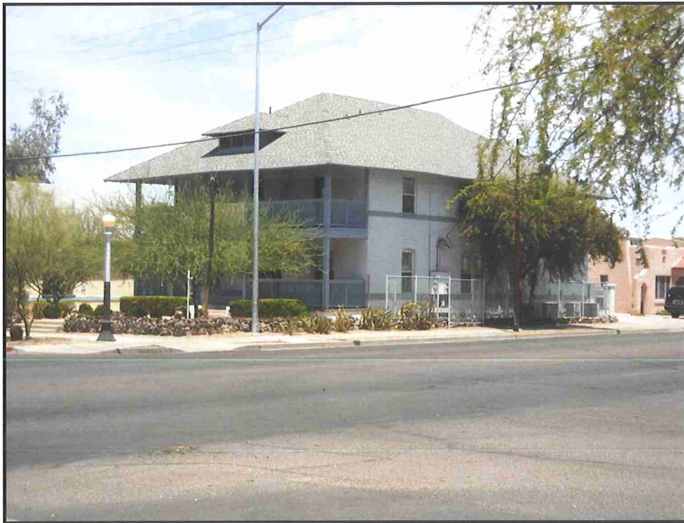
Photograph 11. Carter's Hotel Rest Sanatorium, view facing northwest (2010).
