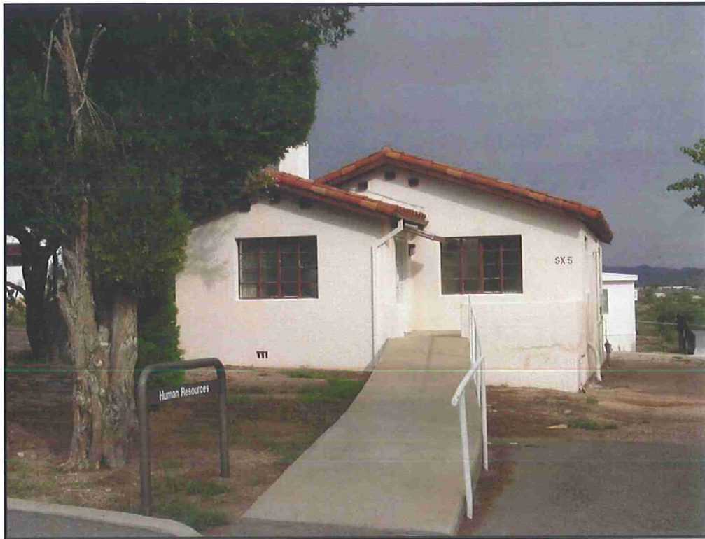
Photograph 41. Former physician residence (San Xavier-5), view facing northwest (2010).
