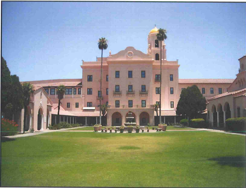
Photograph 26. Veteran's Administration Hospital No. 51, interior courtyard of main building, view facing east (2010).
