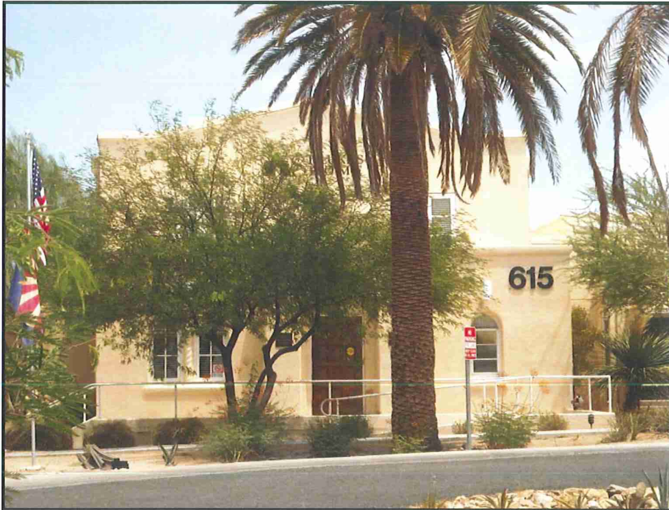
Photograph 7. St. Luke's-In-The-Desert, main administration building, view facing north (2010).
