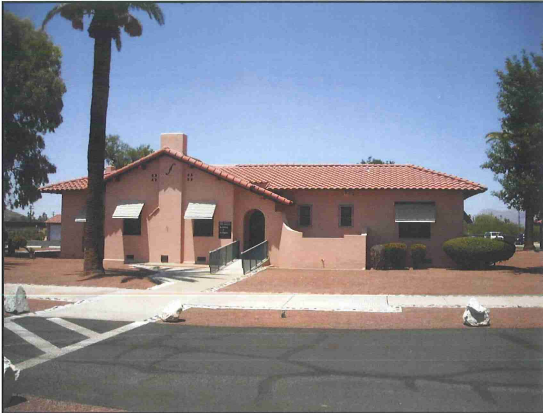
Photograph 29. Former doctor's residence (one of 6 similar residences; three of which exhibit the same plan), at Veteran's Administration Hospital No. 51, view facing north (2010).
