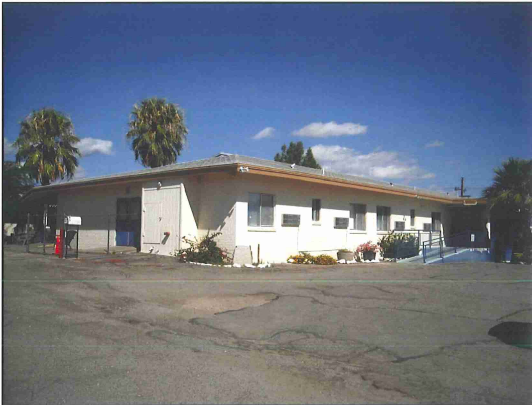
Photograph 56. Main hospital building at the former Arizona State Elk's Association Hospital, view facing northwest (2010).
