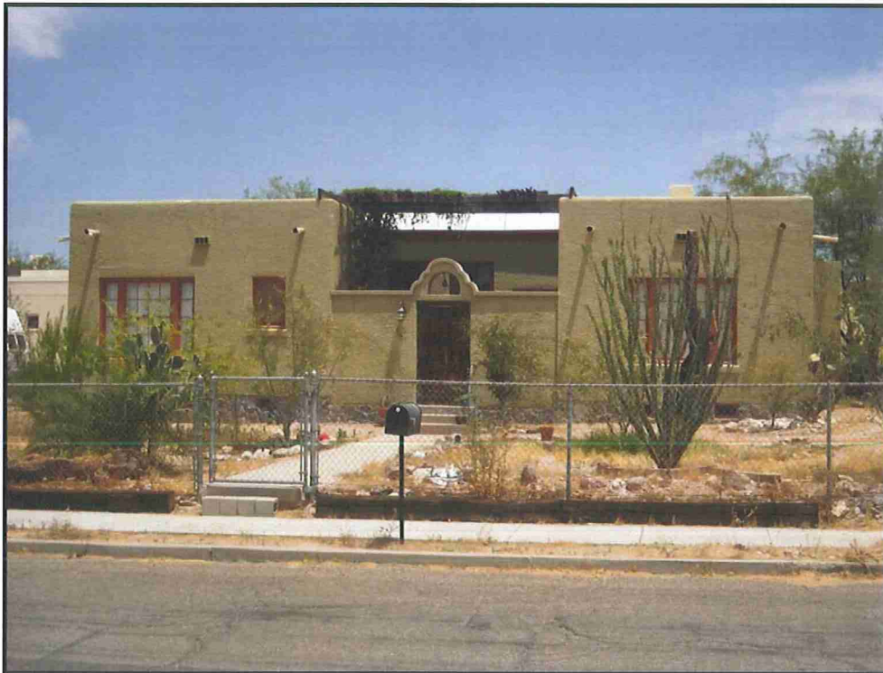
Photograph 9. Former superintendent's residence at St-Luke's-In-The-Desert, view facing north-northwest (2010).
