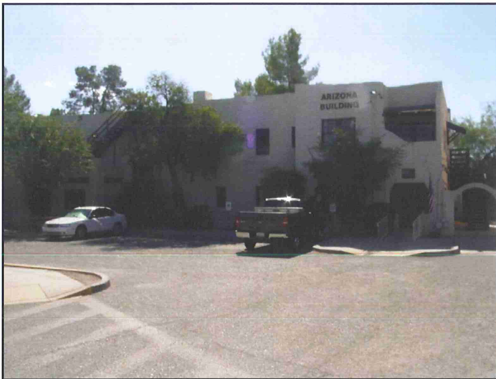
Photograph 18. East elevation of the Arizona Building (nurse's residence) at the former Desert Sanatorium (now Tucson Medical Center), view facing west-southwest (2010).
