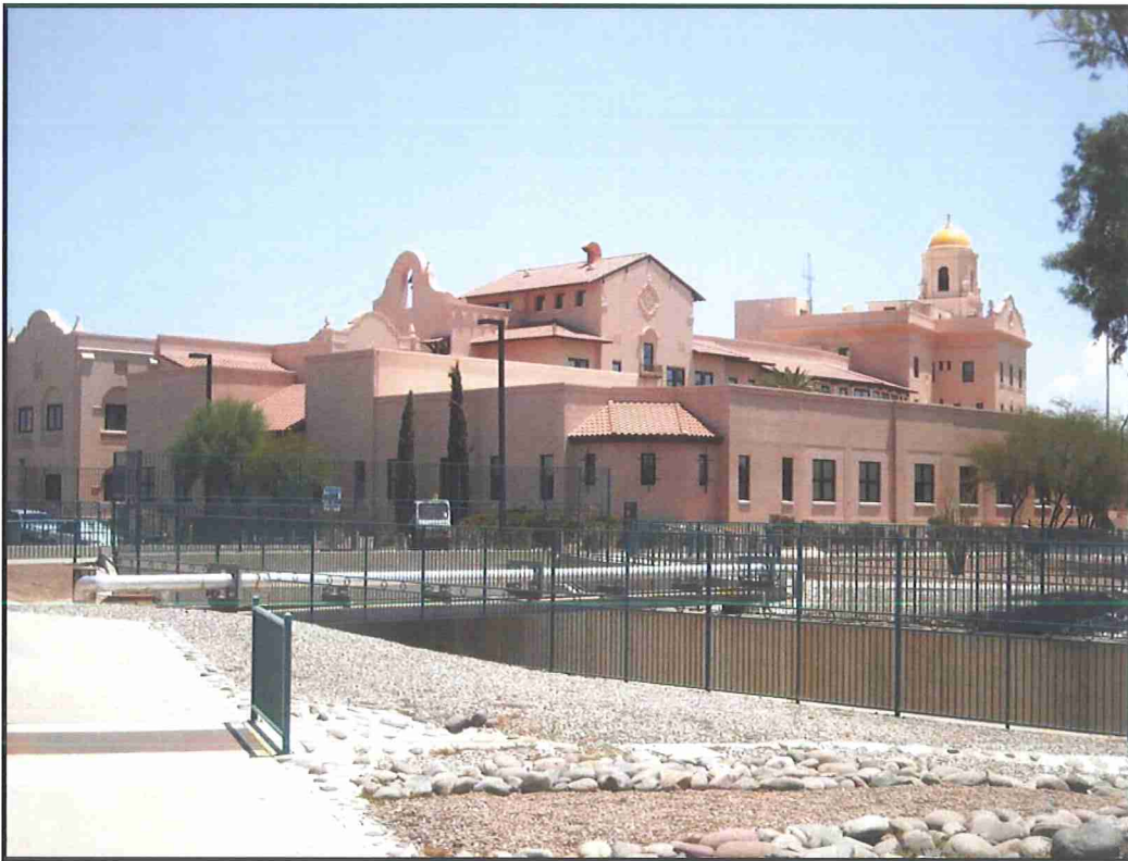
Photograph 25. Veteran's Administration Hospital No. 51, main building, view facing southeast (2010).
