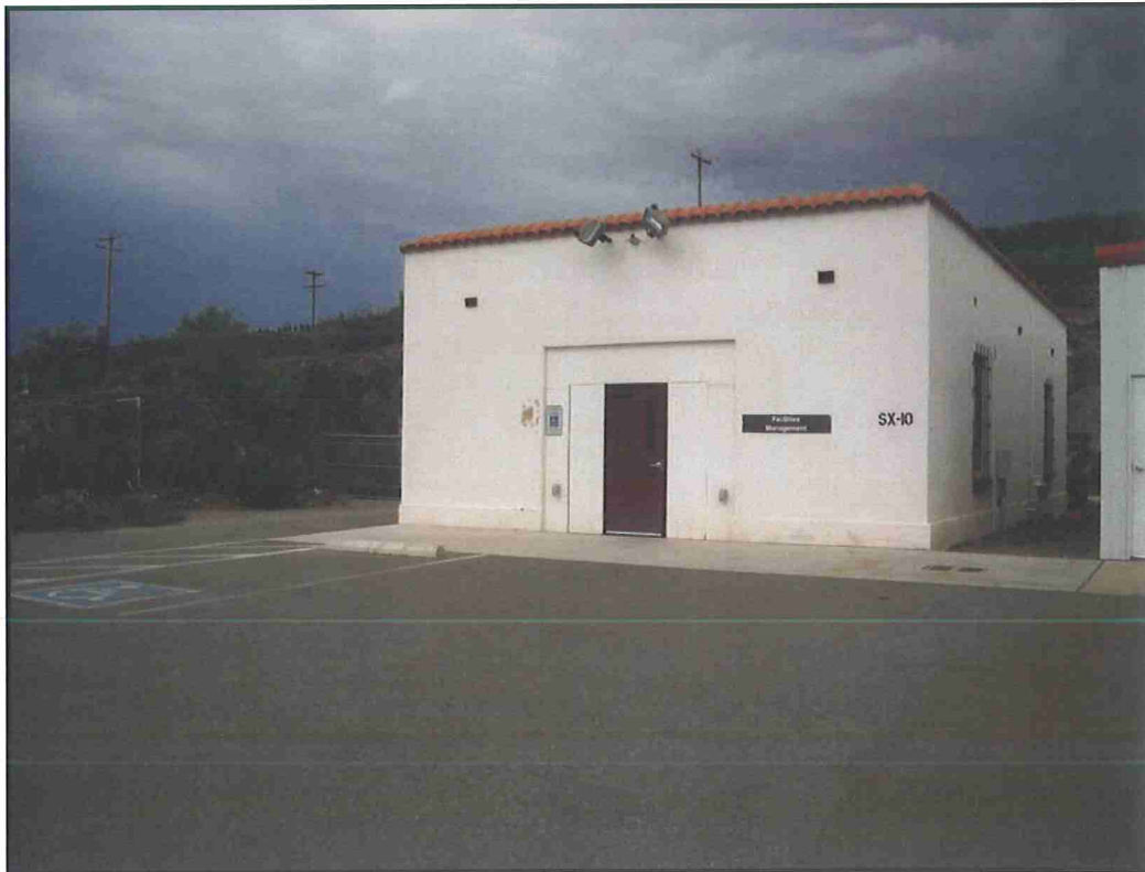
Photograph 45. Former custodial/maintenance warehouse (San Xavier-10), view facing southeast (2010).
