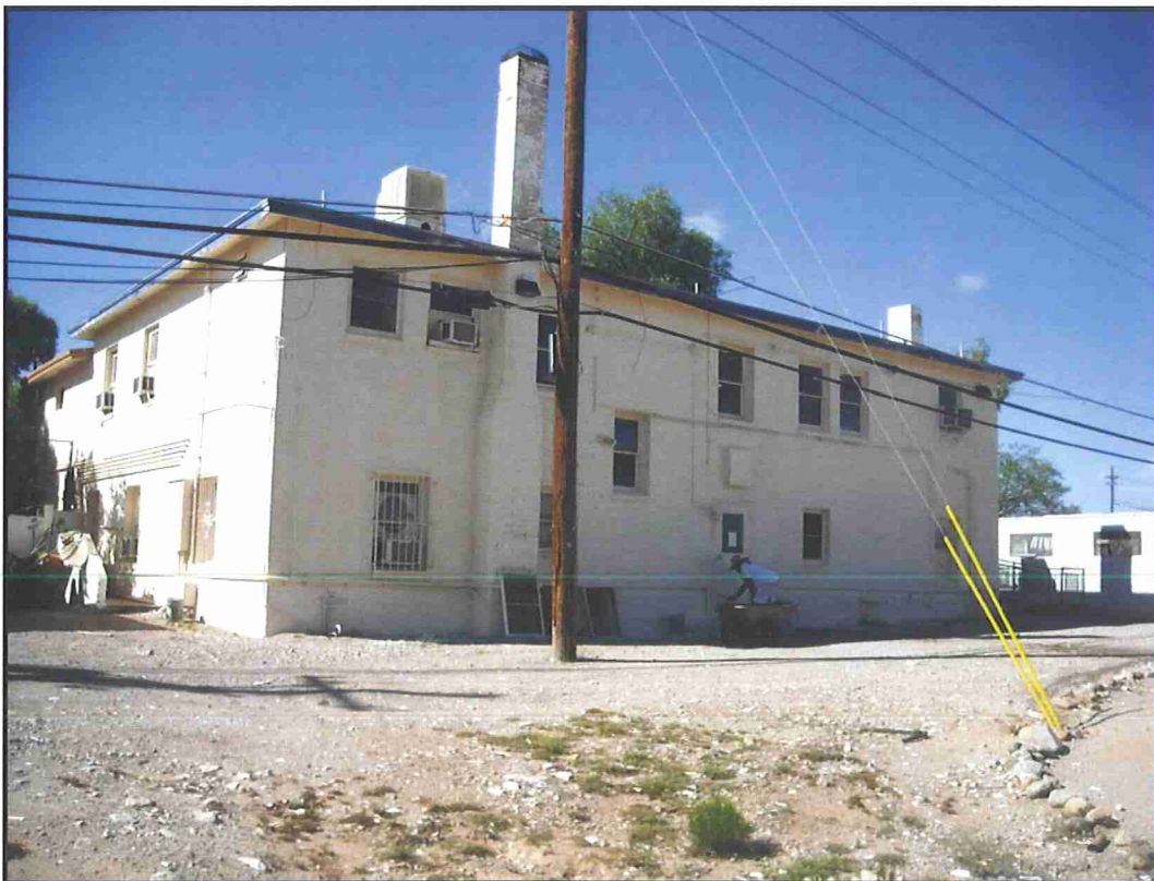
Photograph 57. Former patient ward and incinerator at Arizona State Elk's Association Hospital (near northeast corner of building), view facing southwest (2010).
